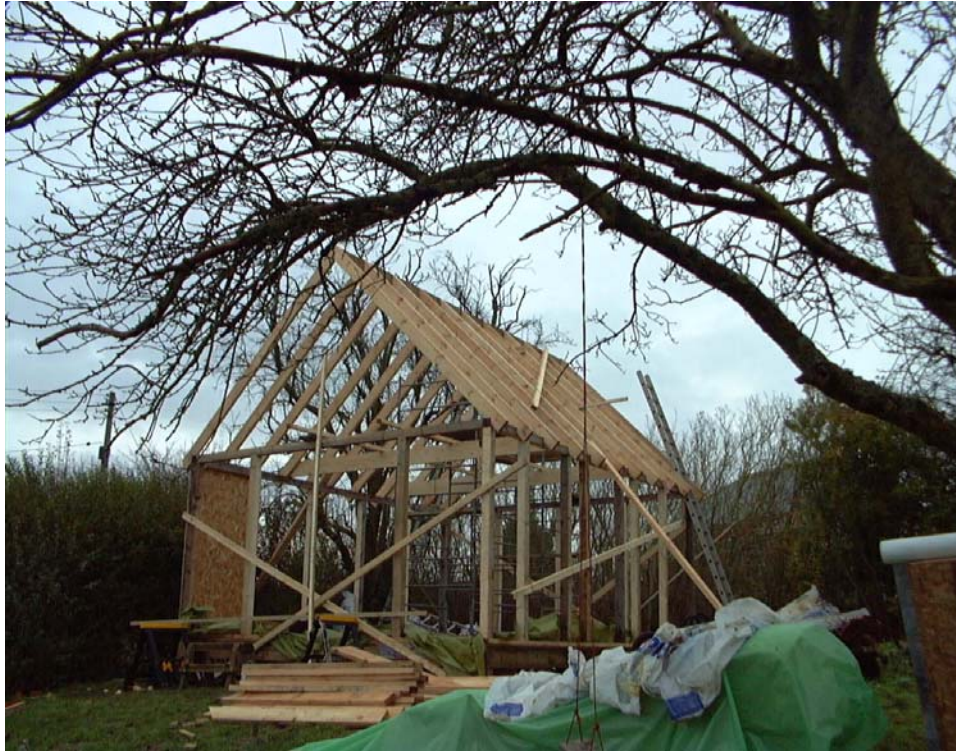
Post and beam barn being built
